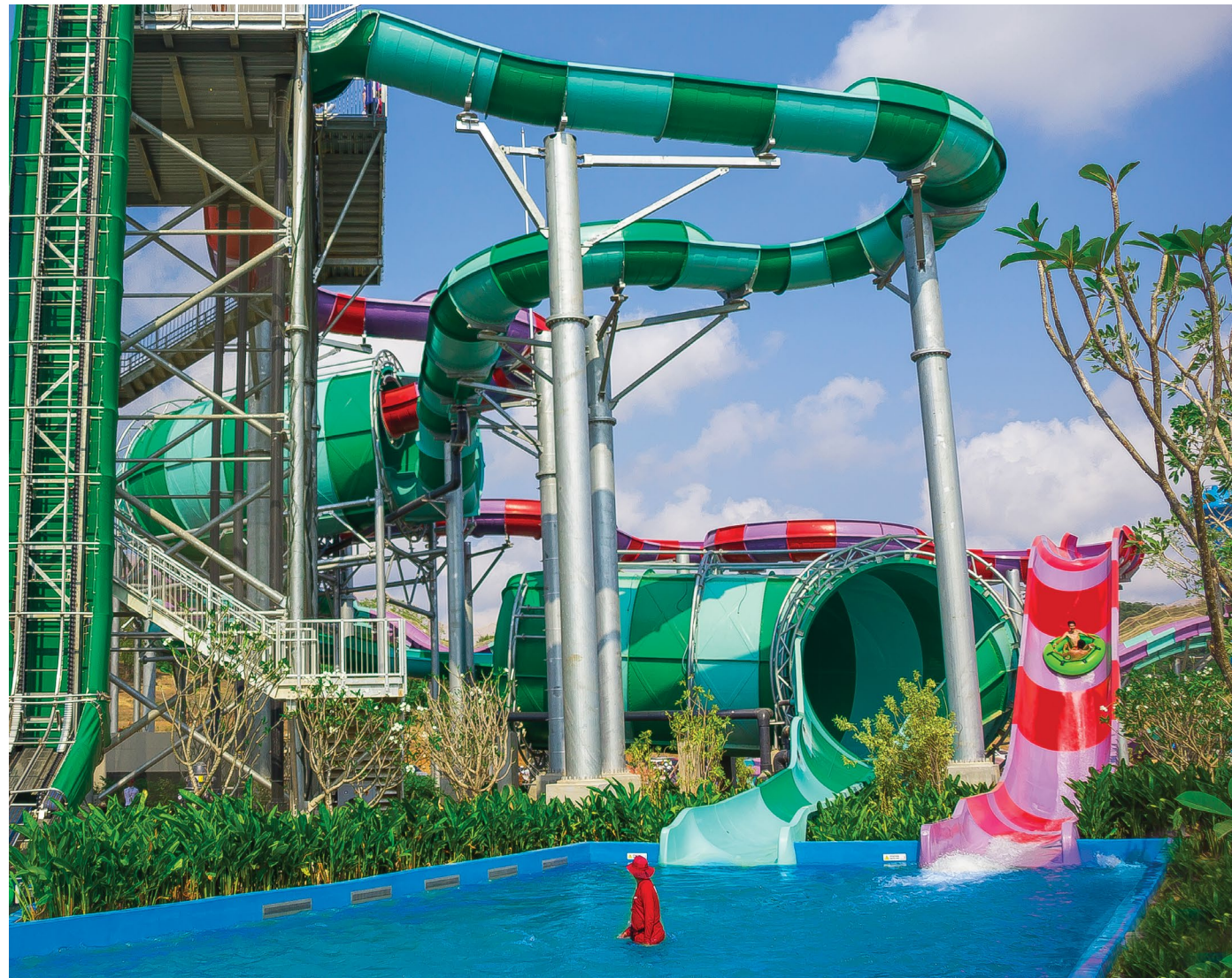
Ramayana Water Park - Chon Buri, Thailand
