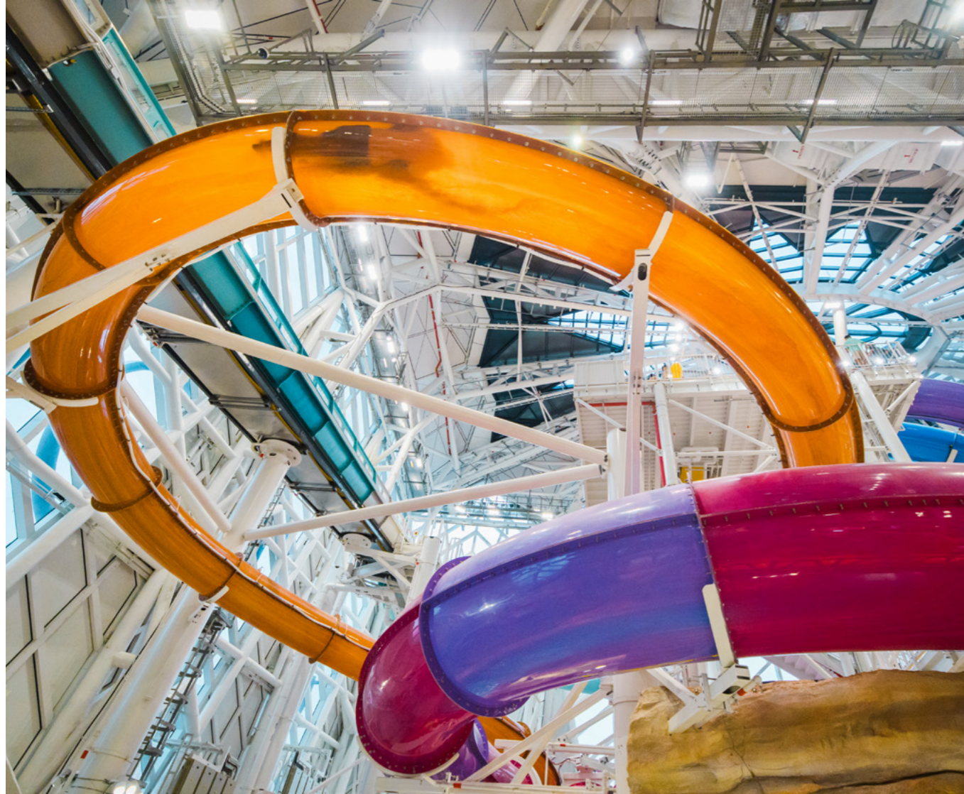
Flatline Loop (Studio City Water Park - Macau, China)
