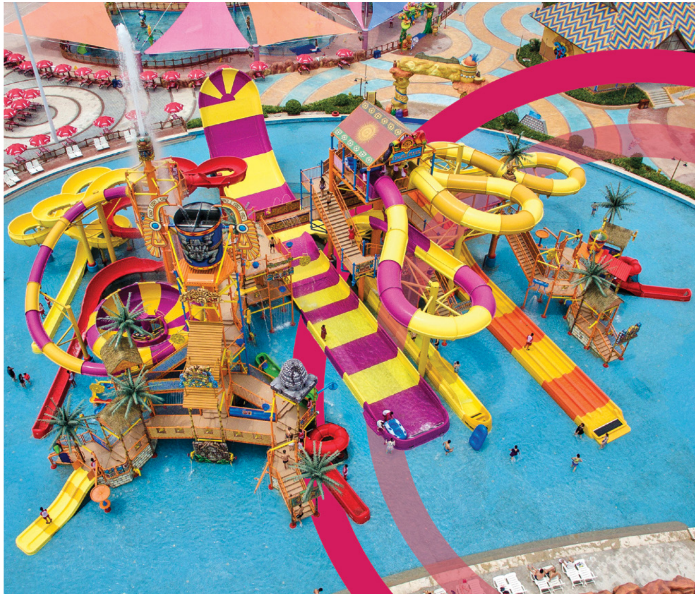
FusionFortress 17 (OCT Playa Maya Water Park Tianjin - Tianjin, China)
