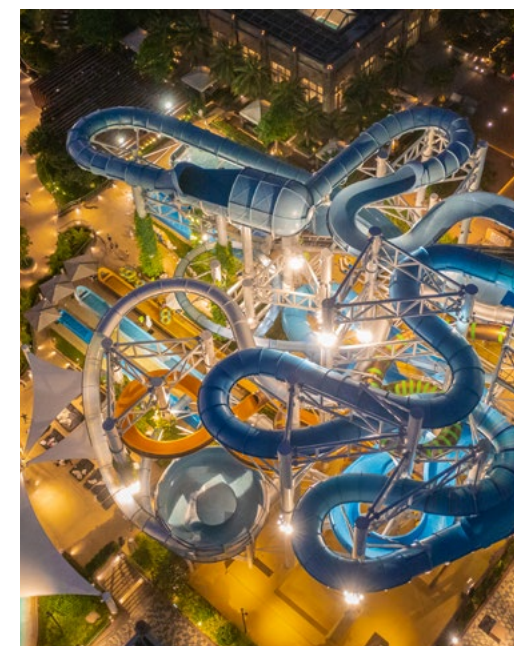
Slide Tower (Studio City Waterpark - Macau, China)
